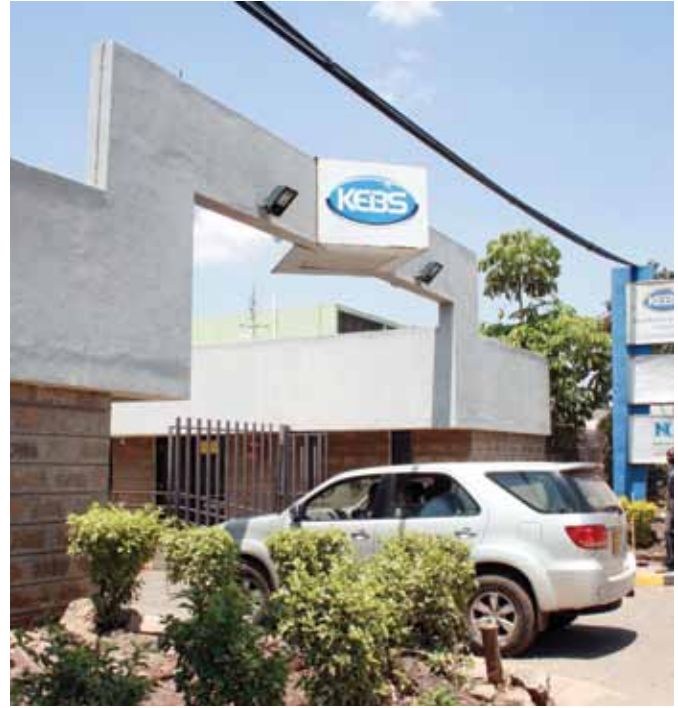
Kenya Bureau of Standards headquarters – Nairobi
